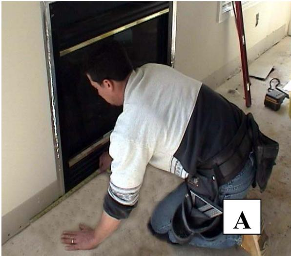
4. **A.** Measure and mark off the area around the firebox to determine where the hearth is going to fit on center. This will provide the area in which to lay the thin set. Following the "thin set" or mortar instructions, spread the mortar so that it extends to all the corners. Using a 3/8" trowel, trowel out the mortar allowing it to fully support the hearth. **B.** Lay hearth. **C.** Shimming should not be necessary using thin set.
