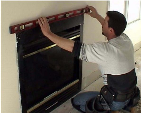
1. Ensure the fireplace is installed plumb and level. The face flushes with the outer surface of the wall. Correct any problems before proceeding. (It is a good practice to inspect the top of the firebox for trash or other combustible materials and remove them.)
