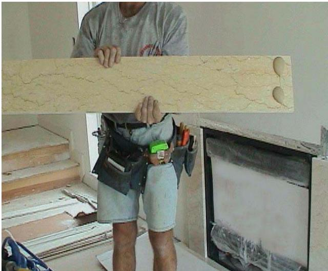
6. Apply silicone adhesive in 4 places (two at each end) to the back of the header at its outer ends and set it on top of legs. Pull back for 30 seconds and re-position header.
