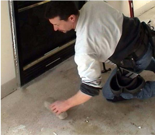
3. Make sure that the floor area in front of the fireplace is level and clean, and has minimal flex. Correct any problems before proceeding. **(For wood-burning applications, a thermal break will need to be laid prior to hearth installation. "Micor" or "Wonder board" is recommended. See fireplace manufactures recommendations.**
